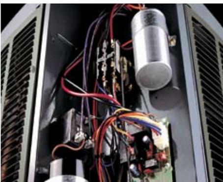
Every Trane air conditioner and heat pump model is quick to install and service. All electrical and refrigerant controls are always in the same place under one easy to remove corner panel.
